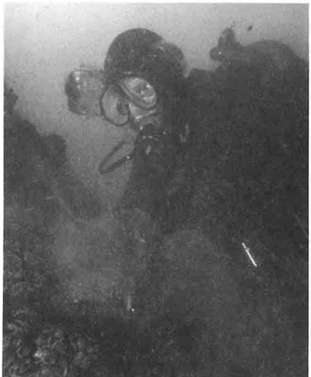
FIGURE 15 Underwater inspector cleaning pile.
