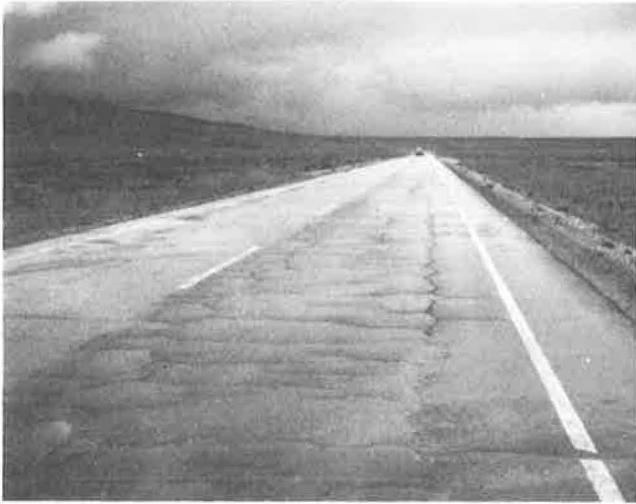
FIGURE 4 Typical transverse cracking.
