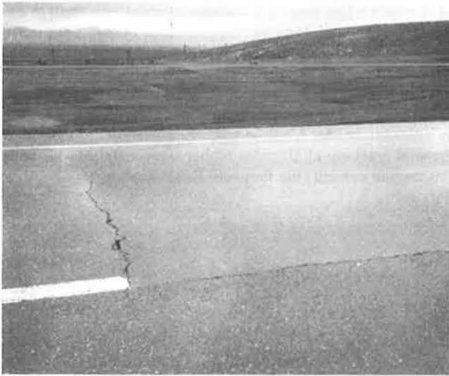
FIGURE 4 Typical transverse cracking.
