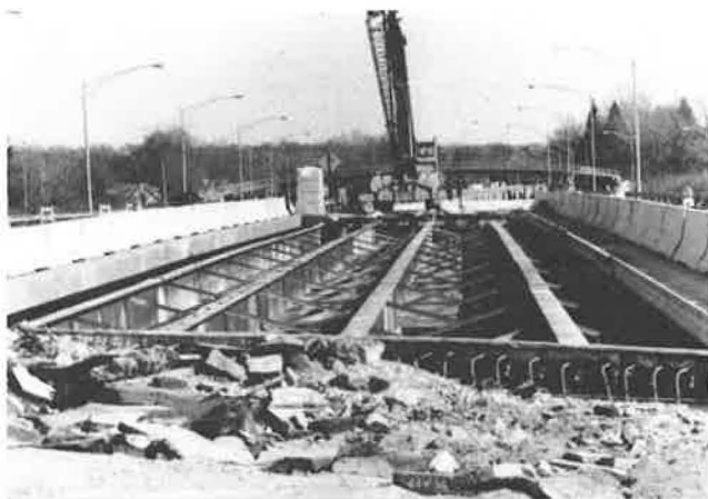
FIGURE 8 Beam lines with deck removed.
