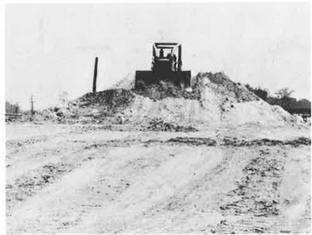
FIGURE 3 Placement of surcharge.
