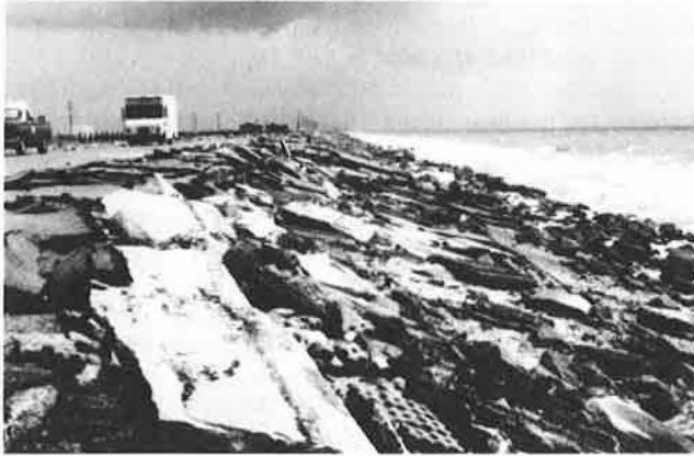
FIGURE 1 Left: A section of LA-82 after tropical storm Chris in 1982, and Right: one of the several revetment projects along LA-82.
