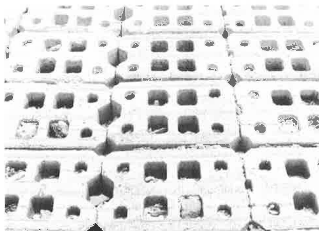
FIGURE 8 Type D revetment.
