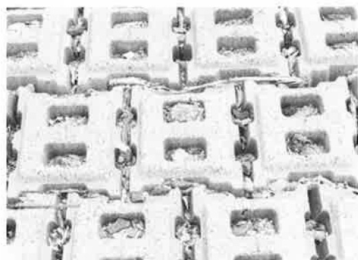
FIGURE 7 Type C revetment.
