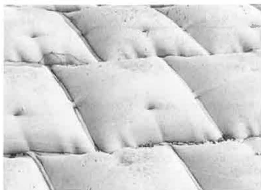
FIGURE 11 Type F cast-in-place cellular concrete revetment.
