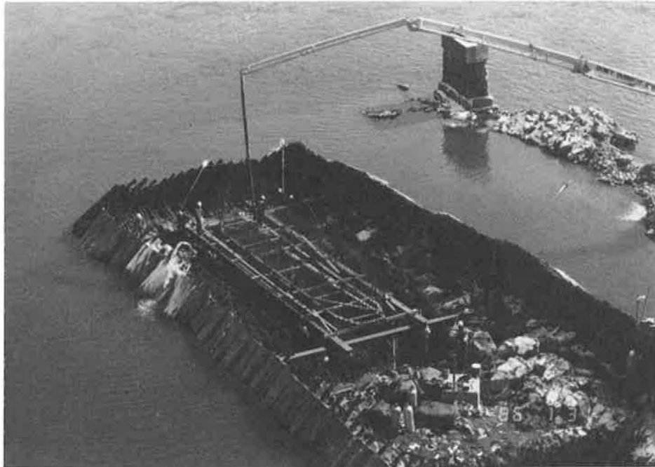
FIGURE 3 Placing of pier concrete in footing with protection of cofferdam.
