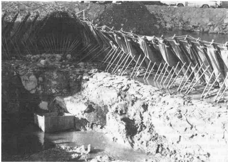
FIGURE 2 Fabric cofferdam on steel frames after rock blasting.
