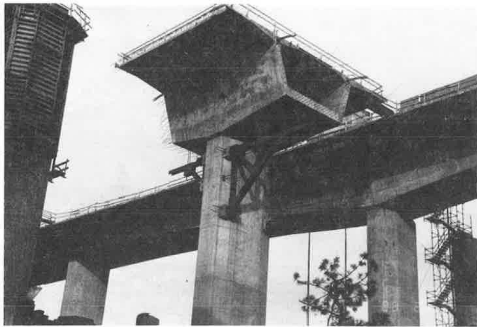
FIGURE 4 Pier table (two-web) with brackets awaiting traveler erection.
