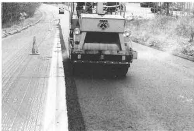
FIGURE 9 Rolling the mat at the wedge edge.
