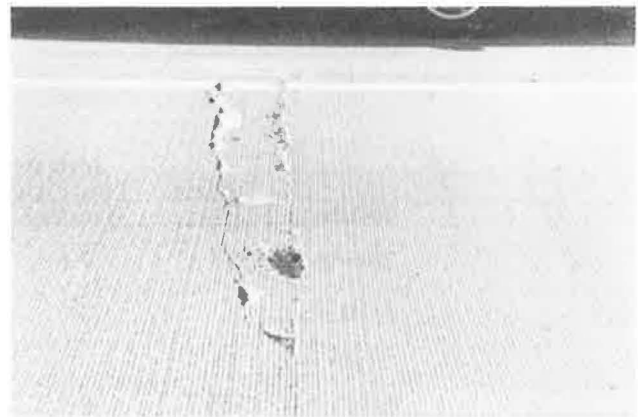
FIGURE 5 Type 2 spalling, I-39.
