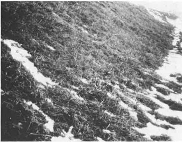
FIGURE 9 Maryland Route 410 project photo.
