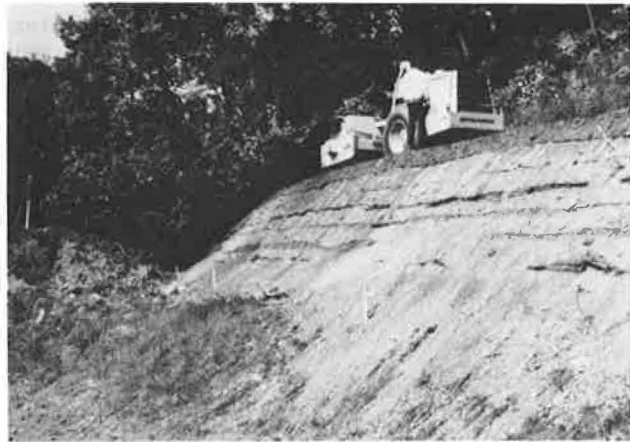
FIGURE 3 Surficial reinforcement on a 1:1 fill.
