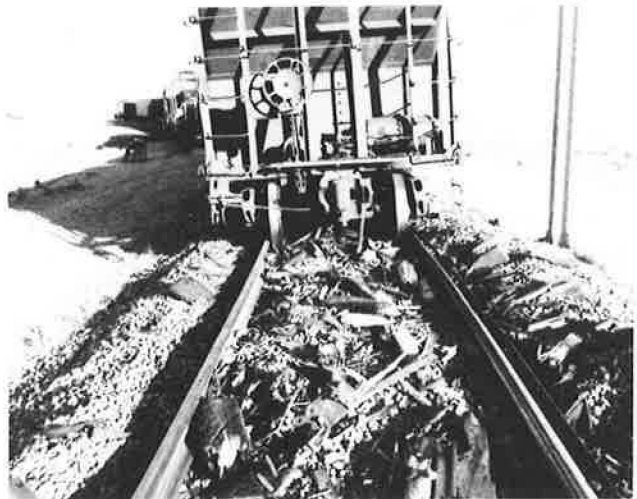
FIGURE 20 Last car derailed.
