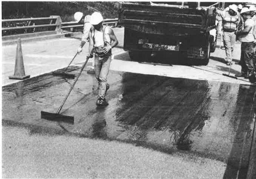
FIGURE 5 An epoxy urethane mixture is here spread over the deck with notched squeegees. Basalt aggregate is here broadcast to excess from the back of a dump truck. Polymer overlays constructed with epoxy, polyester, methacrylate, and epoxy urethane can be used to increase the skid resistance of bridge decks.
