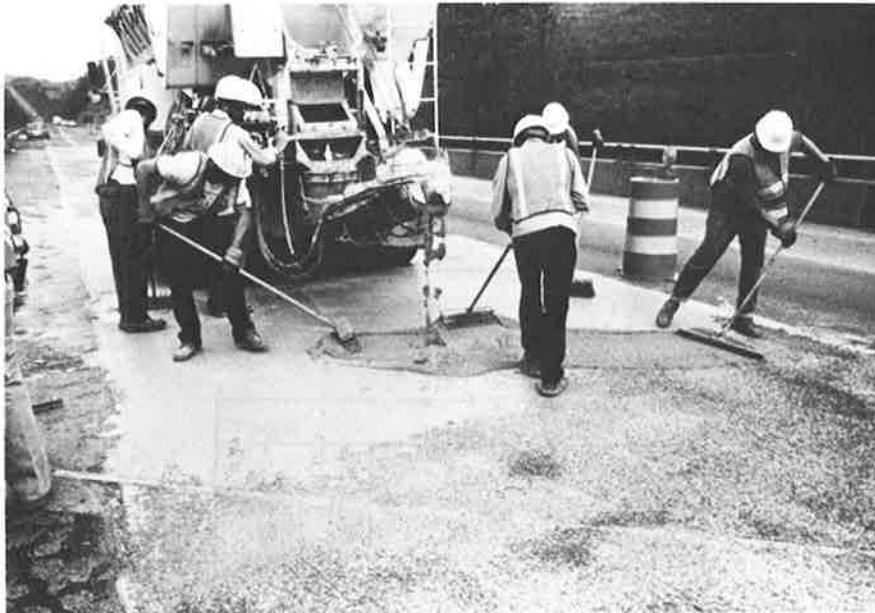
FIGURE 4 A latex modified slag slurry overlay is here applied to a bridge deck to increase the skid resistance. Brooms should be used to brush the slurry into the shot-blasted surface and the slurry should be struck off and pulled forward with gage rakes set to provide a 3/16 in to 1/4 in thick slurry. For increased skid resistance slag should be broadcast onto the struck off surface, and a liquid curing material should be applied to prevent the evaporation of water. The slurry can be opened to traffic in two to three days.
