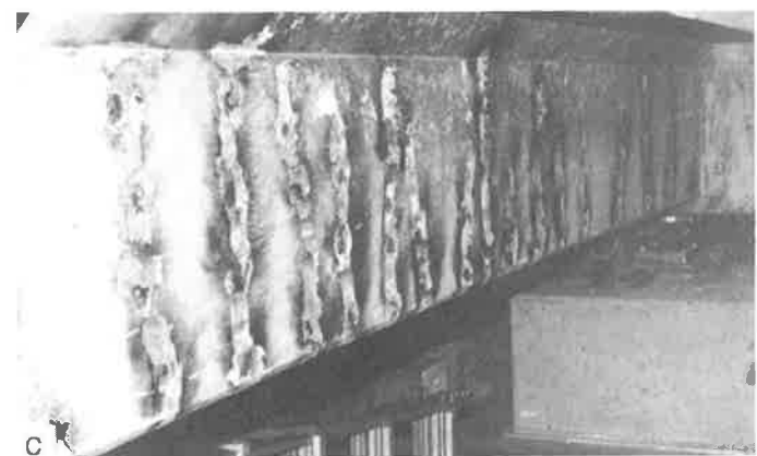
FIGURE 3 Epoxy injection of flexural cracks
