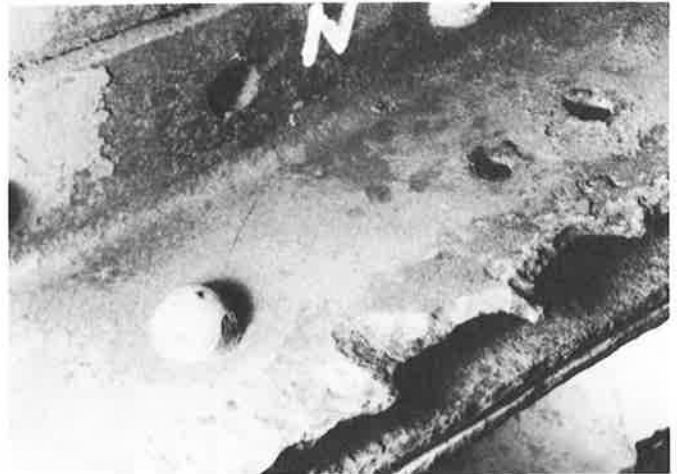
Figure 9 Corrosion Pitting of Beam Flange and Welded Coverplate
