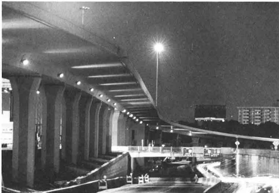
Figure 10. San Antonio "Y". Completed Project IIIA&B at night. Lighting for at-grade facility was provided by fixtures embedded in the elevated structures.
