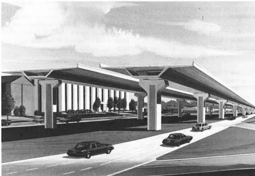
Figure 12. U.S. 183, Austin, Texas. Twin parallel structures 58' wide each are used to produce this 1.25 million square foot bridge.
