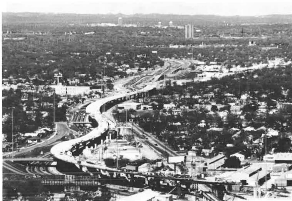
Figure 6. San Antonio "Y". Aerial view of IIIA&B Project. Second-level bridges are placed within existing right-of-way. All aspects of highway geometry are accommodated in span-by-span precast segmental construction.
