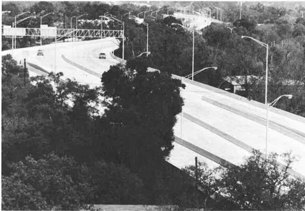
Figure 4. Biloxi, I-110. As many as four precast box girders were used side-by-side to provide the total bridge deck width.
