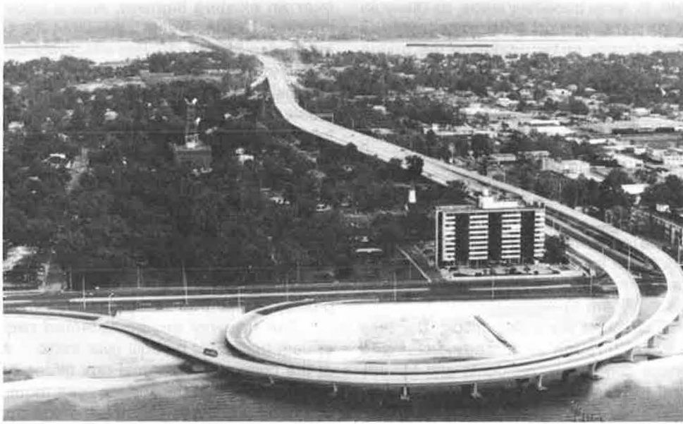
Figure 1. Biloxi, I-110. Aerial view of completed elevated structure.
