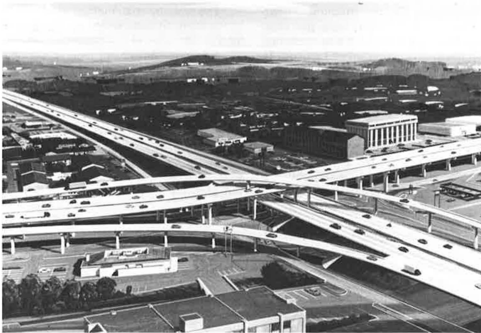
Figure 11. U.S. 183, Austin, Texas. Aerial view of Interchange of 183 and IH-35. Direction ramps at 4th level are built in cantilever. Main lanes at 2nd or 3rd level are built in span-by-span.
