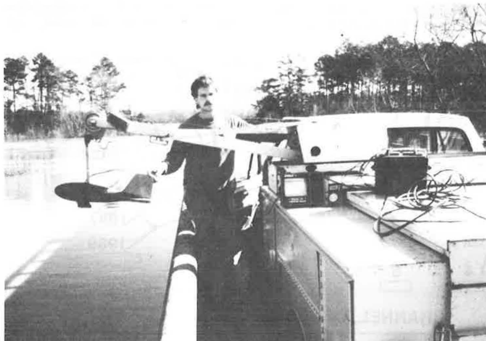
Figure 8. Truck-mounted crane used to suspend and manipulate the weight over the side of the bridge.
