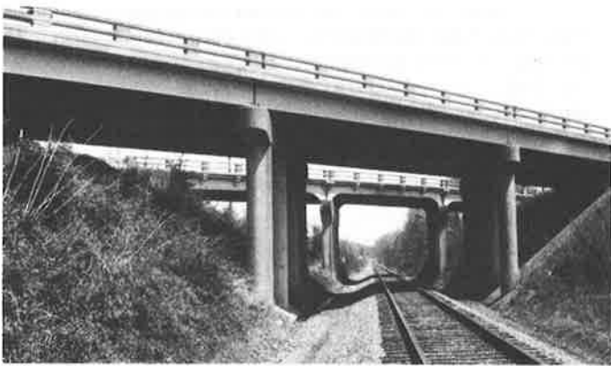
FIGURE 2 Photograph of 3 span skewed concrete bridge
