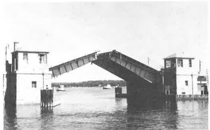
FIGURE 1 Bayville Bridge. A view of bascule span.
