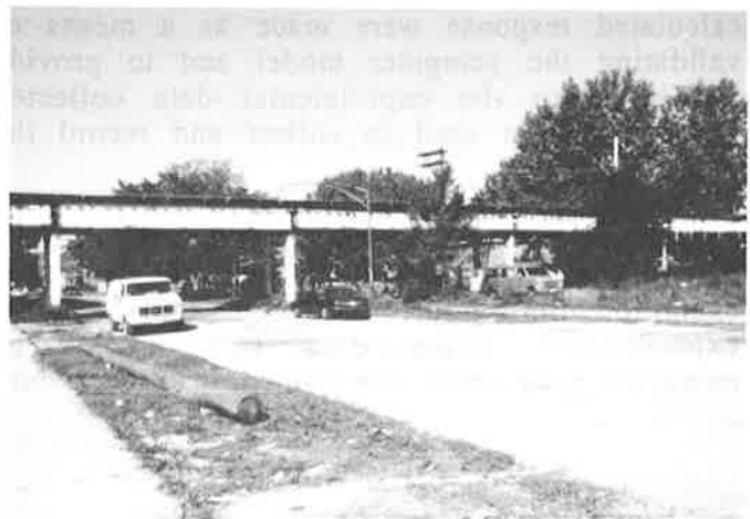
Figure 1. View of Elevated Structure, Test Span Left of Center
