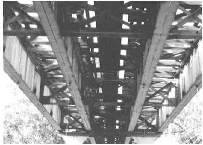
Figure 4. View from Below Test Span Structure
