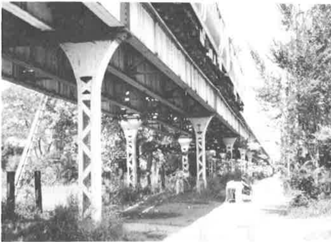
Figure 3. View of Static Load Test
