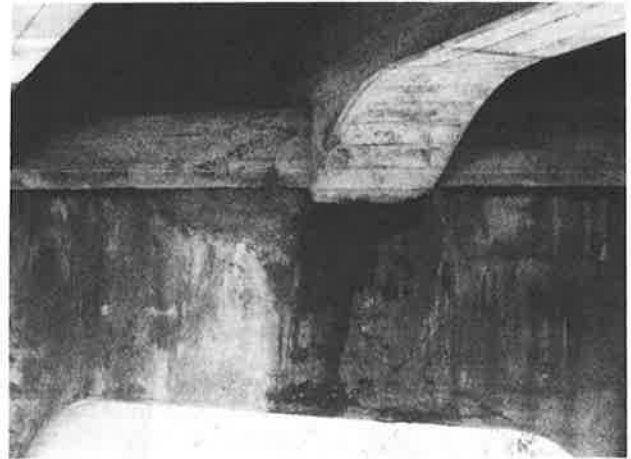
FIGURE 3 Repaired spalled concrete bridge piers
