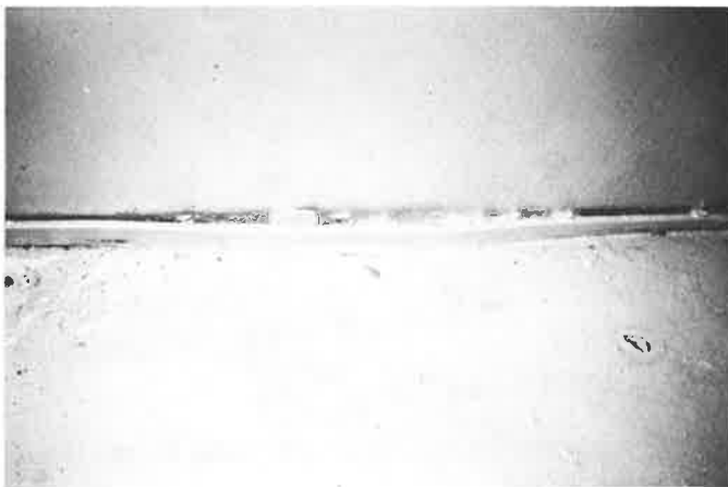
Figure 11. Backing Bar Inside Box Cap Member is Bent Away from Cap Web
