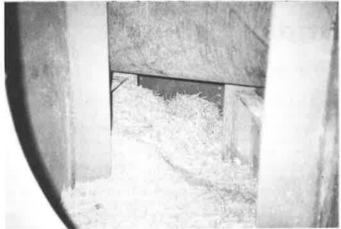
Figure 24. Nesting Material Inside Box Cap Member
