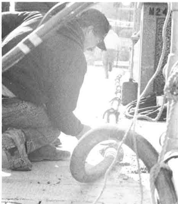
FIGURE 9 Two-inch hose for pumping concrete.
