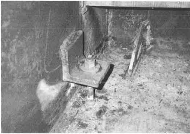
Figure 8. Angle and Bolt Welded to Inside of Box Cap Member
