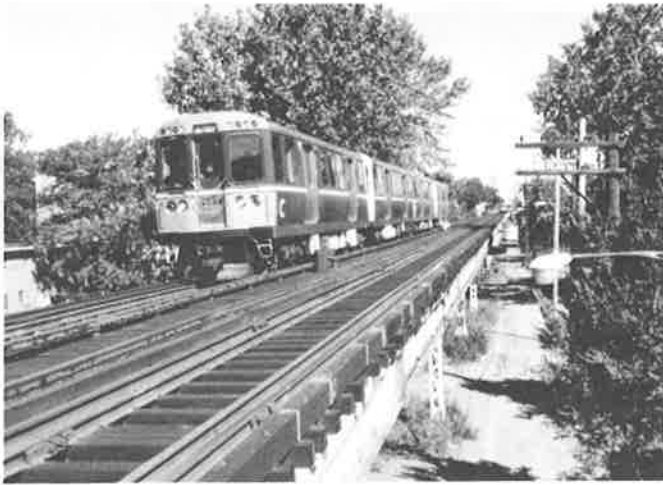
Figure 2. View of Tracks Along Test Area
