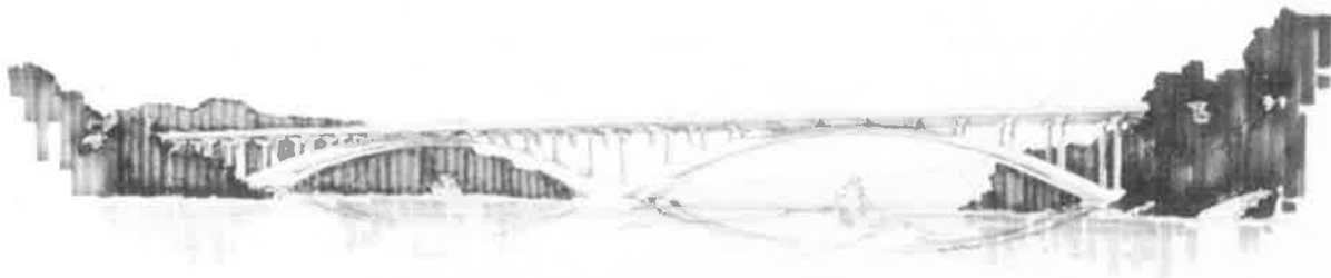
FIGURE 1 Rendering of two-ribbed concrete arch bridge.
