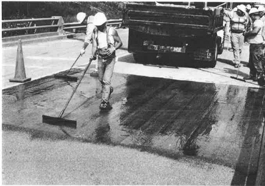
FIGURE 5 An epoxy urethane mixture is here spread over the deck with notched squeegees. Basalt aggregate is here broadcast to excess from the back of a dump truck. Polymer overlays constructed with epoxy, polyester, methacrylate, and epoxy urethane can be used to increase the skid resistance of bridge decks.
