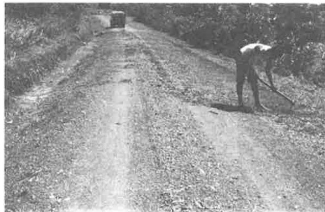
FIGURE 6 Grubbing edge.
