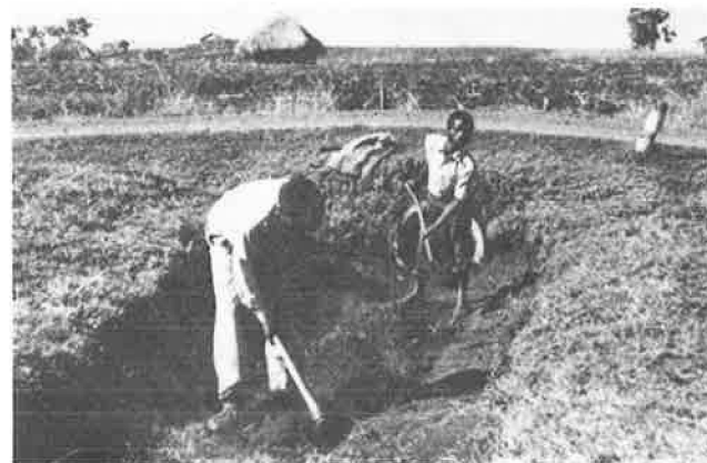
FIGURE 9 Cleaning culvert outlet.
