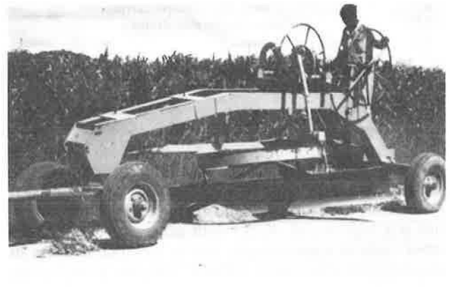
FIGURE 12 Towed grader under trial.
