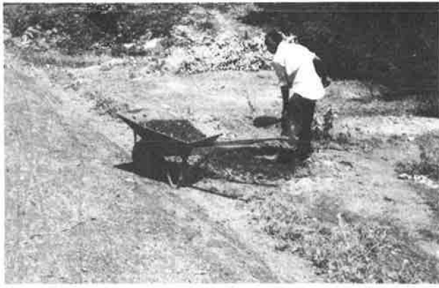
FIGURE 7 Excavating gravel for patching.
