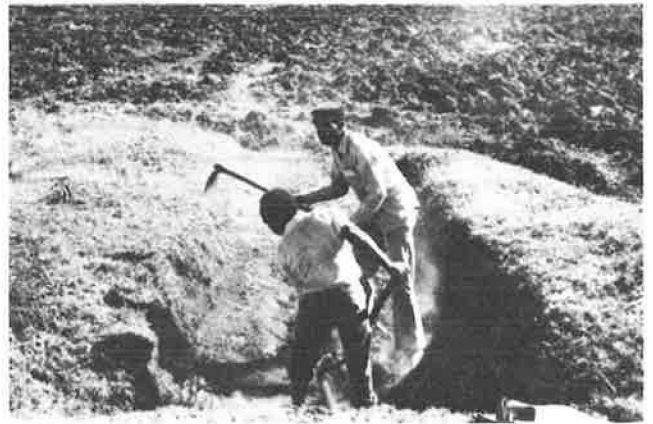
FIGURE 10 Cleaning culvert inlet.
