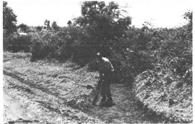
FIGURE 11 Cleaning miter drain.
