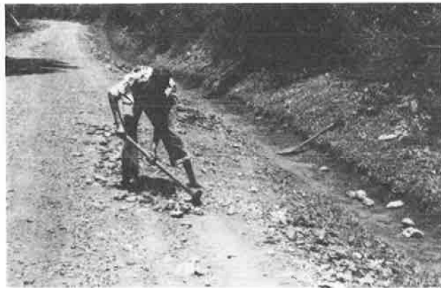
FIGURE 8 Reshaping carriageway.
