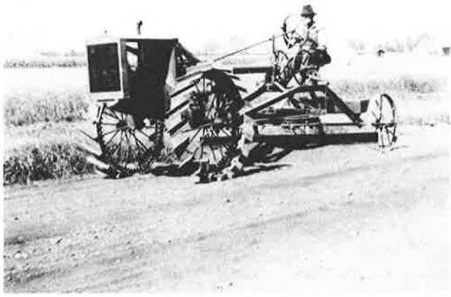
FIGURE 1 Self-propelled grader, 1919.
