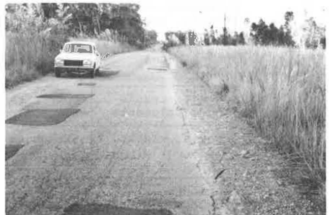
FIGURE 4 Wide ruts resulting from traffic consolidation of a lateritic boulder pavement on a lateritic plateau (National Road 4, Tampoketsa Plateau, Madagascar).
