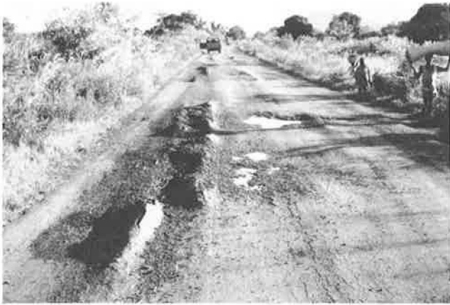
FIGURE 5 Narrow ruts and longitudinal heaving resulting from weathering of a basaltic natural gravel (National Road 5B, near Sambava, Madagascar).
