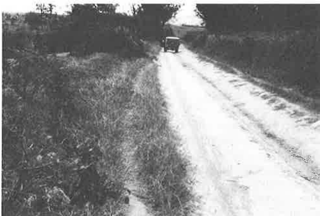
FIGURE 6 W cross section, Kilometer 10 from northern end, National Road 44, Madagascar; the hollow segments of the cross section are particularly sharp as a result of wearing by iron fellies of bullock carts.
