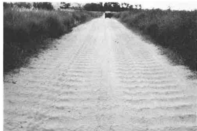
FIGURE 8 Corrugations of a lateritic gravel pavement, road Kelo to Moundou, Chad; W cross section is also apparent.
