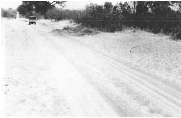
FIGURE 10 Rutting of dry cohesionless sand, Kilometer 131, National Road 35, Madagascar.
