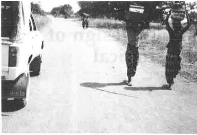
FIGURE 1 A section of the road Lai to Doba, Southern Chad: the pavement material is undisturbed ferruginous soil and the traffic comprises heavy vehicles for collection of cotton crops and transport of miscellaneous goods. A sample of pavement soil was classified as low-plasticity clay, CL, after laboratory testing and exhibited a soaked CBR of 40 percent at 95 percent modified compaction.
