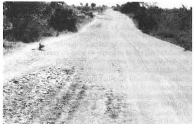
FIGURE 13 Holes and shearing, Kilometer 35, National Road 10, Madagascar.
