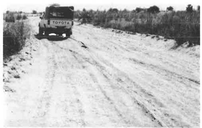
FIGURE 12 Dusty surface of fine soils, Kilometer 55, Kelo-Lai road, Chad.
