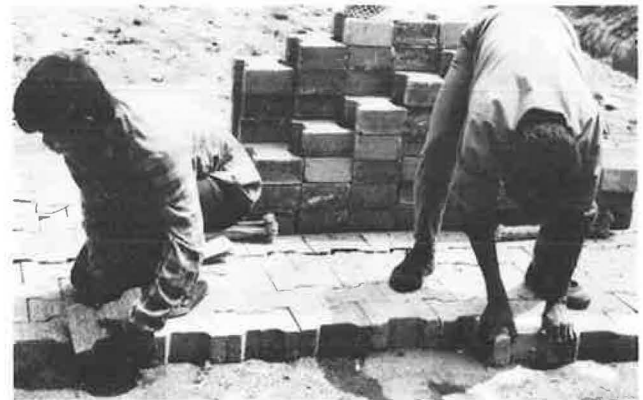
FIGURE 7 Laying concrete blocks.
