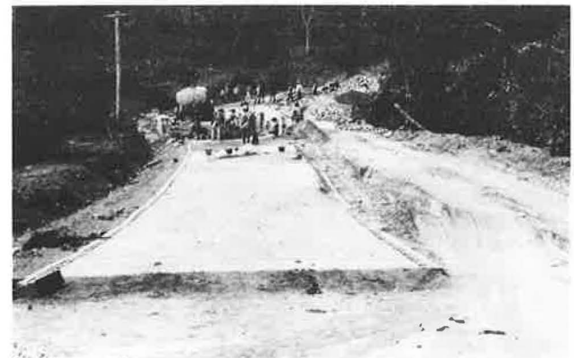
FIGURE 8 Completed lane of concrete blocks.
