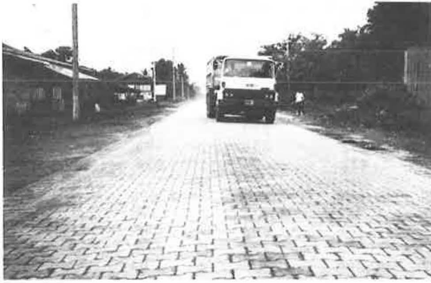
FIGURE 5 Heavy traffic on block pavement.
