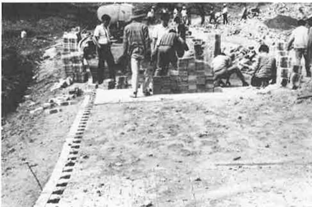
FIGURE 4 Concrete block pavement on steep gradient.
