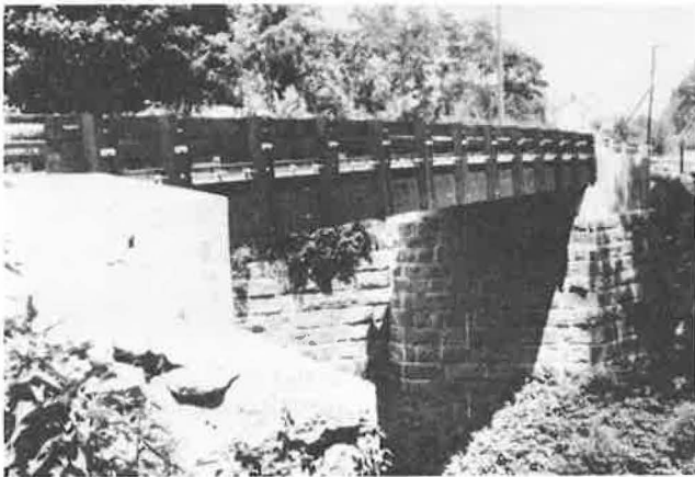
FIGURE 4 Charleston, West Virginia, stressed T-section timber bridge, 73-ft span.
