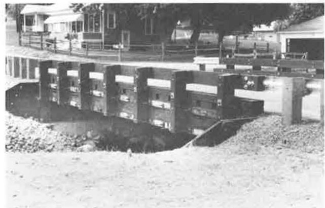
FIGURE 7 Stressed boxed-girder timber of Field Crest Bridge, Morgantown, West Virginia.
