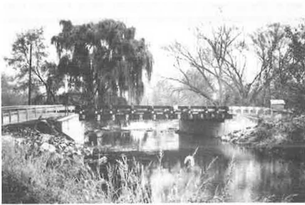
FIGURE 1 Trout Creek Bridge, College Township, Pennsylvania.
