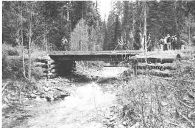
FIGURE 1 Typical log bridge.
