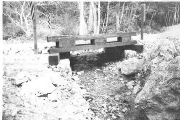
FIGURE 6 Two views of a longitudinal glulam panel bridge.
