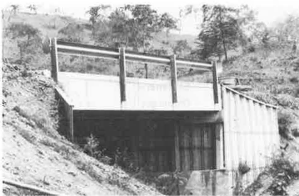
FIGURE 3 Colorado Bridge, Ecuador.
