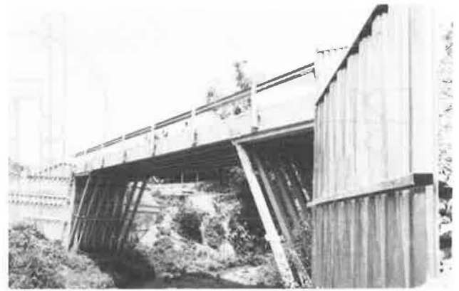
FIGURE 4 Zapallo Bridge, Ecuador.
