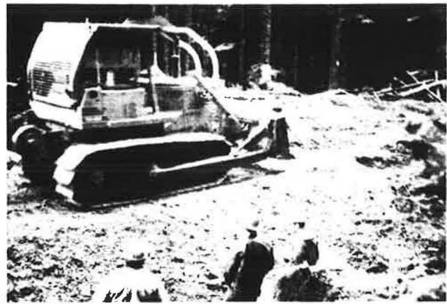
FIGURE 3 Bulldozer used to shape desired road prism.
