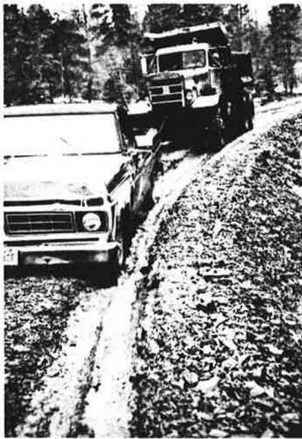
FIGURE 7 Deep ruts resulting from construction haul.
