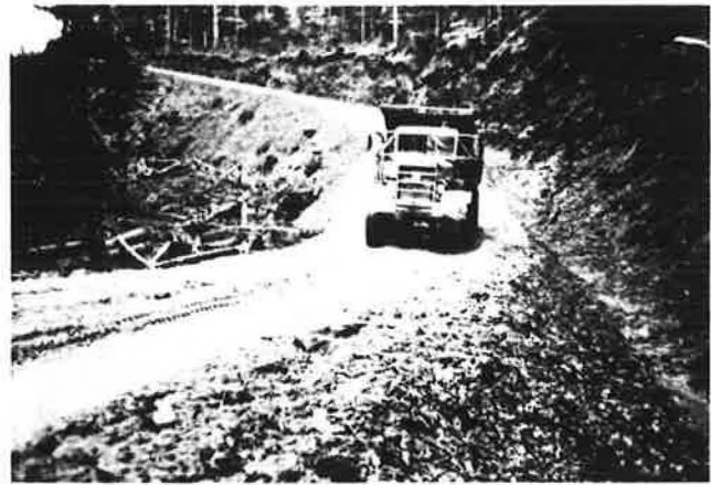
FIGURE 11 Maximum rutting where trucks could not vary wheel path.
