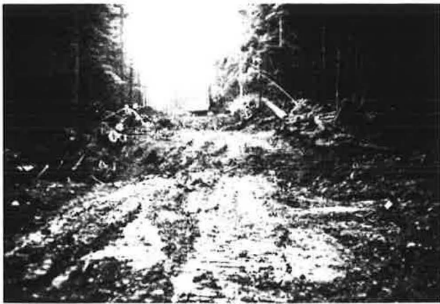
FIGURE 1 Road subgrade preparation.
