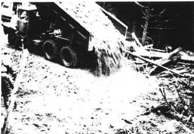
FIGURE 2 End-dumping rock used for road construction.
