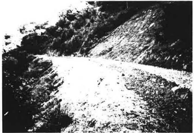
FIGURE 10 Completed fill on Mosquito Ridge Road.
