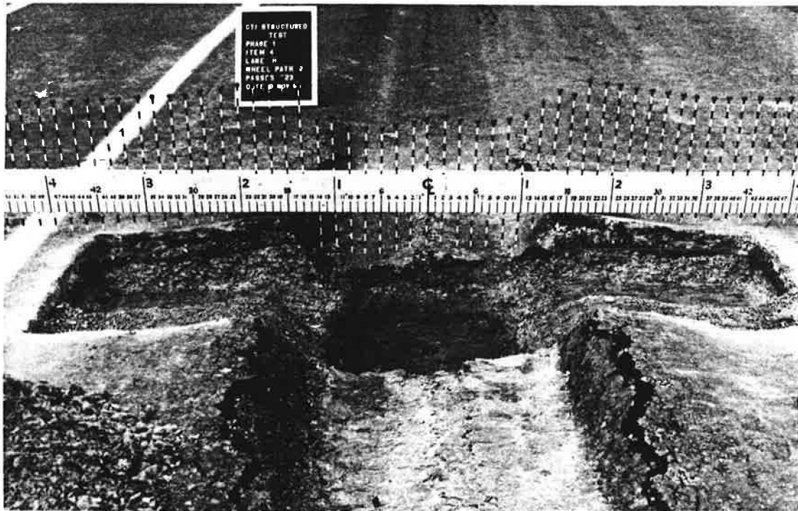
FIGURE 6 High-pressure lane, Section 4, test trench after 323 passes.
