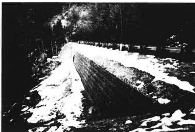
FIGURE 7 Completed wall at Site 17 on Stump Springs Road.
