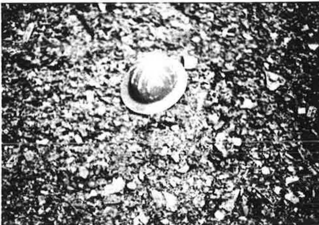
FIGURE 6 Rock borrow after initial placement.
