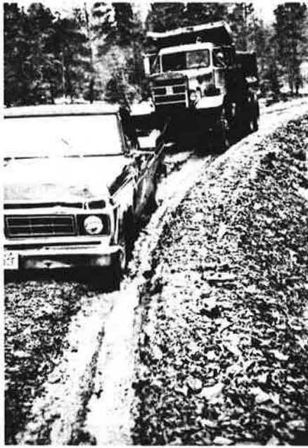
FIGURE 7 Deep ruts resulting from construction haul.
