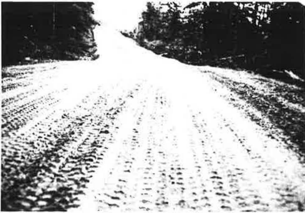
FIGURE 10 Resulting road surface, full-width travel.
