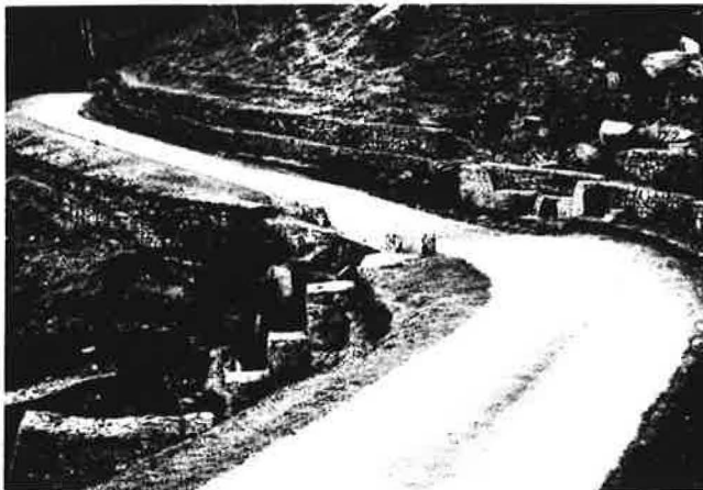
FIGURE 6 Typical causeway for smaller rivulets.
