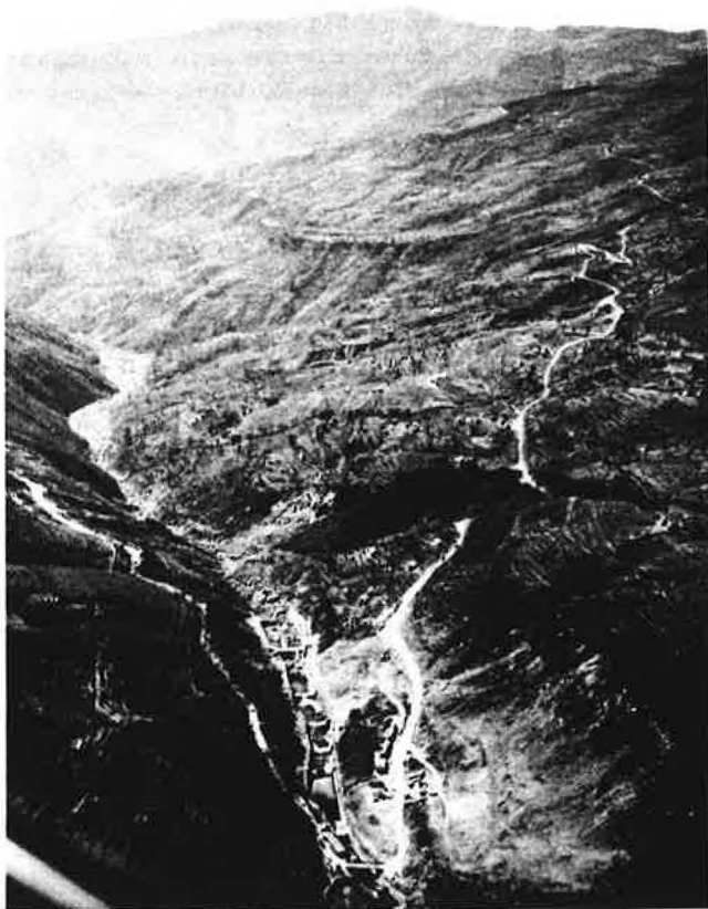
FIGURE 2 Aerial photograph of project area, looking south; Charnawati crossing in the foreground.
