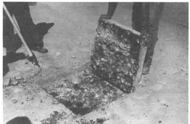
FIGURE 4 Typical pavement sample.
