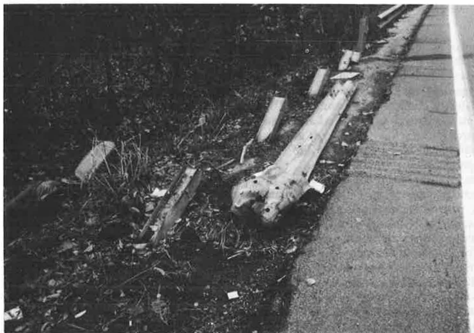
FIGURE 1 Vehicle path and guardrail end in collision: NASS-LBSS Case 83-08-512T.
