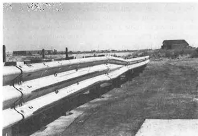
FIGURE 12 Vehicle contact marks, Test 475.
