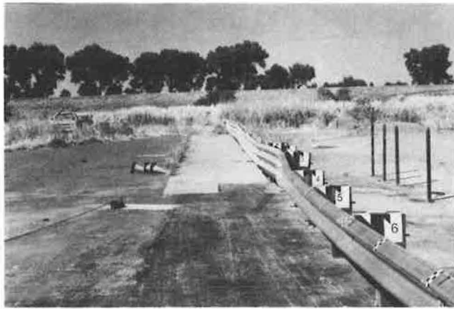
FIGURE 13 Rail damage: displaced posts, bent rail, broken post, Test 475.
