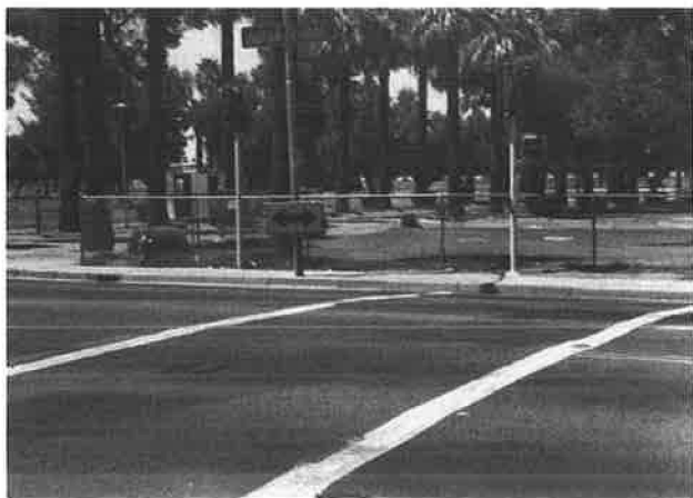
FIGURE 1 Condition of Indian School Road after 19 years.
