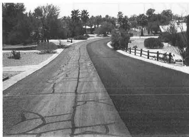
FIGURE 6 Overlay with asphalt rubber hot mix: condition before overlay (left); completed half (right).
