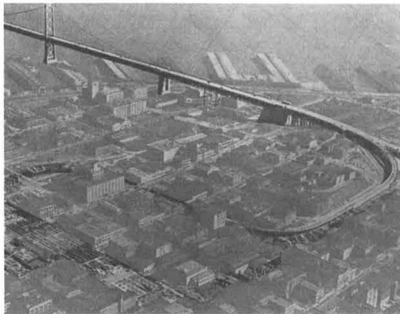
FIGURE 4 Demolition of 34 city blocks for terminal and viaduct construction (3).
