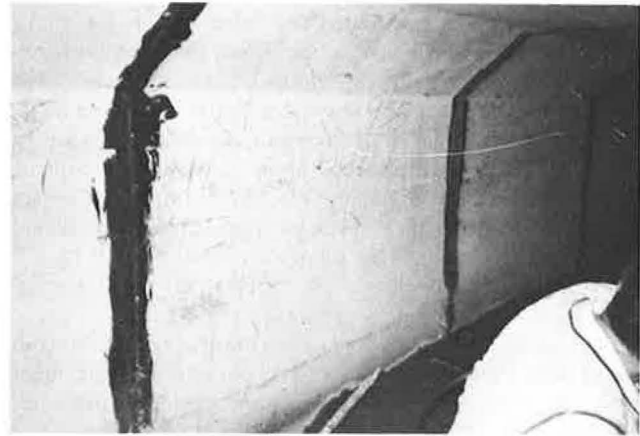
FIGURE 7 Joint material spread on inside of joint.
