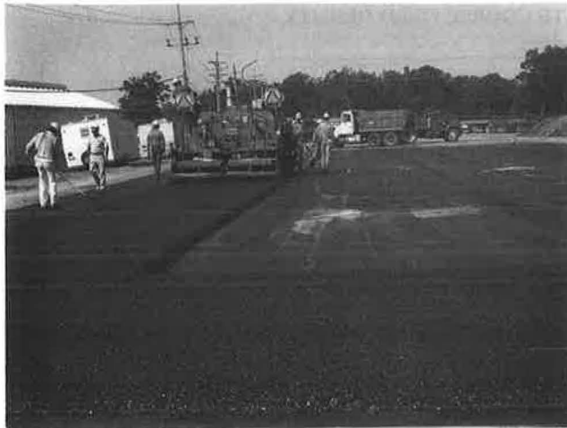
FIGURE 2 Placing open-graded asphalt material.
