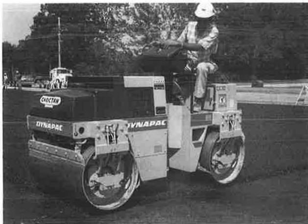
FIGURE 3 Three-ton steel-wheel roller.
