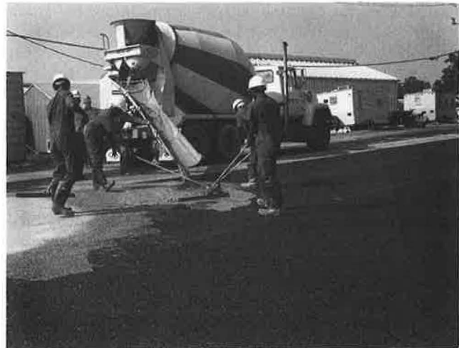
FIGURE 4 Resin-modified slurry grout being applied to open-graded asphalt material.
