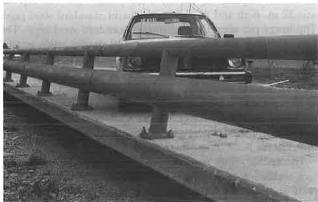
FIGURE 1 T421 bridge rail installation.
