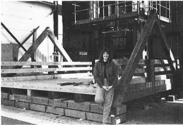
FIGURE 1 18- × 18-ft oak A-frame timber bridge.
