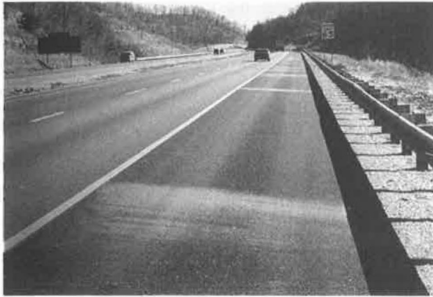
FIGURE 1 Soil-stained shoulders.
