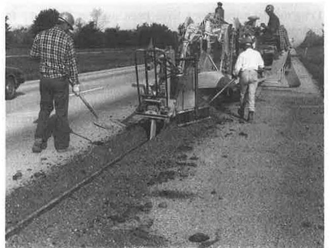
FIGURE 6 Installation of edge drain on I-64, Fayette County.
