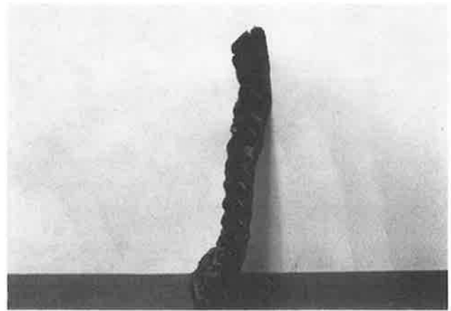
FIGURE 19 Excavated Type-A drain showing compression.
