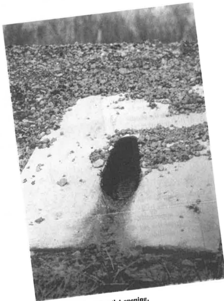
FIGURE 12 Typical outlet opening.
