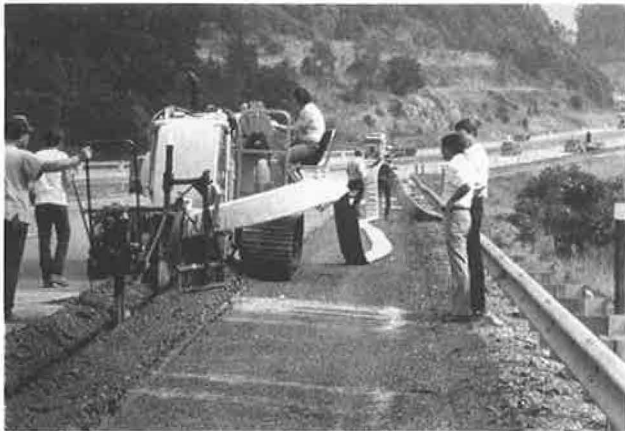
FIGURE 2 Edge-drain installation.
