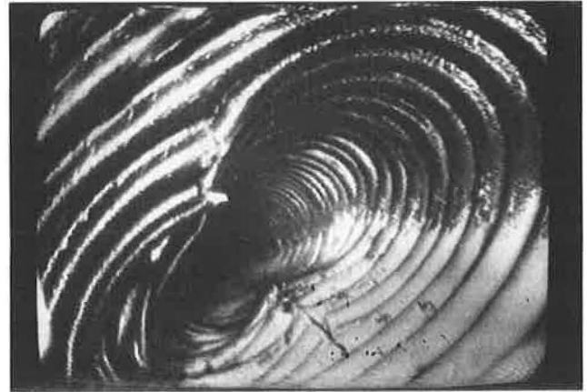
FIGURE 9 Collapsed subdrain.
