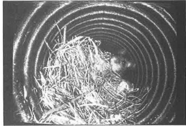
FIGURE 8 Rodent nests in subdrains.
