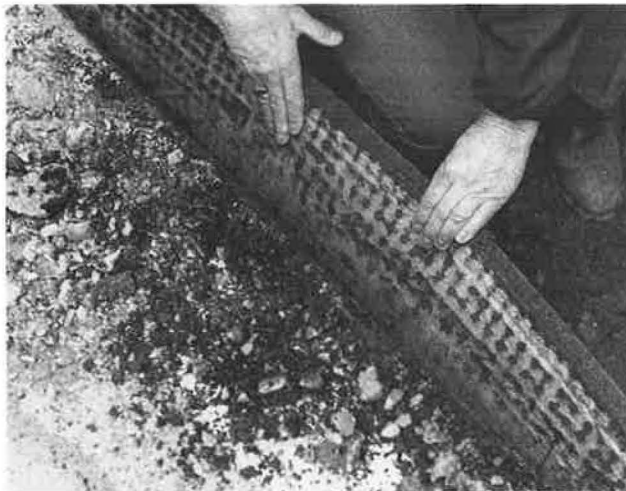
FIGURE 4 Excavated Type-A drain on I-64, Franklin County.
