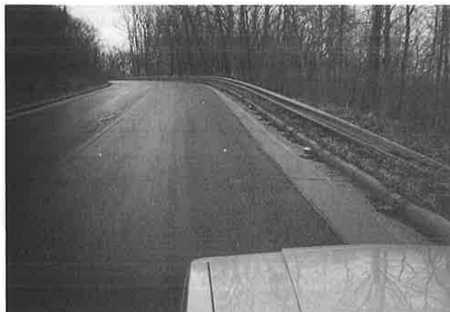
FIGURE 13 Condition of pavement on typical curbed section.
