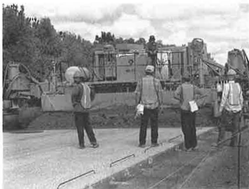
FIGURE 1 Cleaned surface with edge bonding reinforcement bars.
