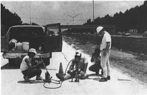
FIGURE 3 ACI pull test was one test used to measure overlay bond strength.
