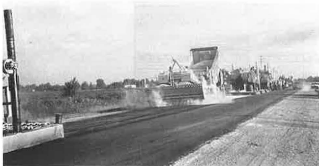
FIGURE 7 Hot manufactured sand being applied approximately 5 mm thick using a chip spreader between the first and second preheater (15).
