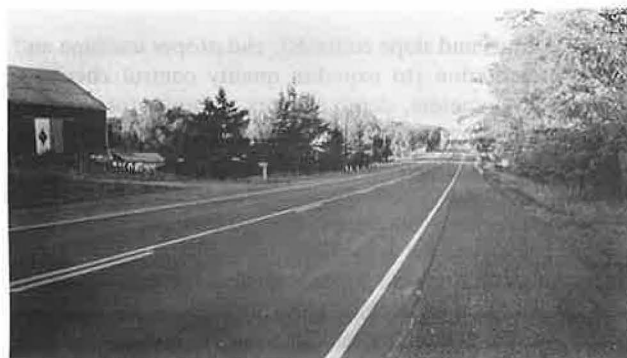
FIGURE 8 Typical rural heat reforming (HRP-5) pavement surface (John Emery Geotechnical Engineering, Limited).
