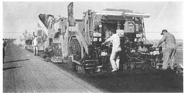
GENERAL VIEW OF HEAT REFORMING PROCESS (HRP-5) AT SPOKANE INTERNATIONAL AIRPORT SHOWING THE TWO PREHEATERS AND REFORMER. The pre-milled (75 mm) keel section involved heater scarification/rejuvenation (50 mm) with new surface course placement (50 mm) in one pass (Remix-Repave Option) [6].
