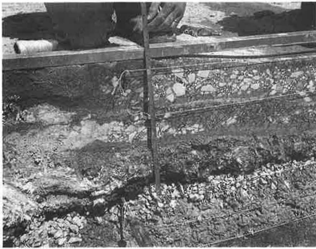
FIGURE 4 Pavement trench at Milepost 17.46, US-23–Louisia Bypass.
