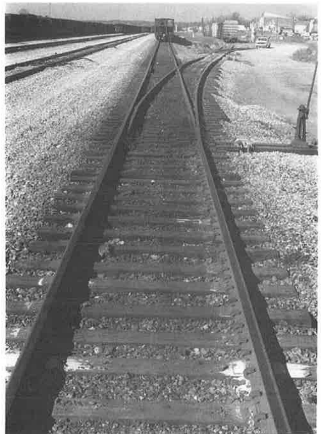
FIGURE 4 CSX Ravenna Yard mainline HMA turnout after 10 years of service.
