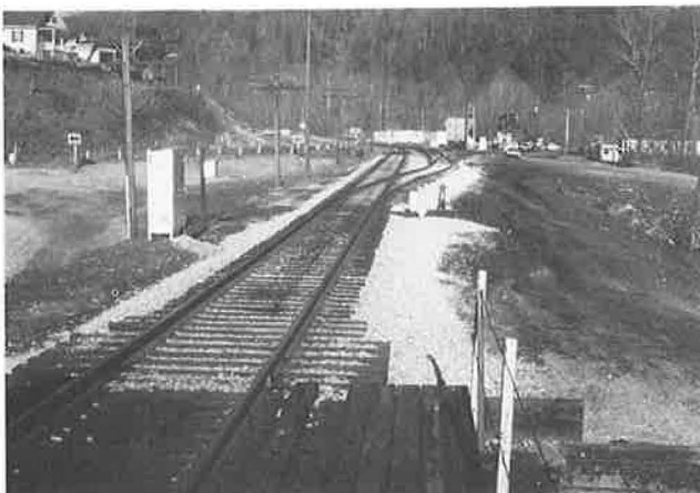
FIGURE 9 CSX Livingston, Kentucky, mainline HMA turnout and bridge approach installation.
