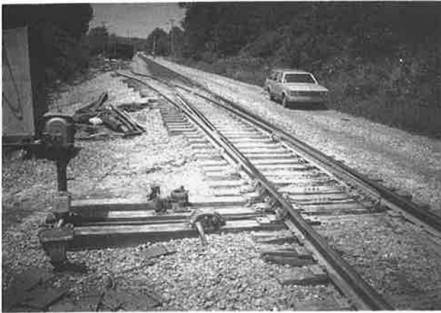
FIGURE 2 Typical pumping turnout before placement of HMA underlayment.
