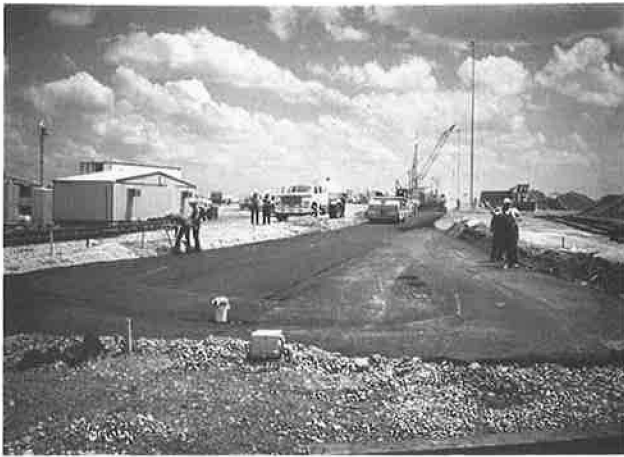
FIGURE 5 Santa Fe Flynn Yard hump track with HMA in place.
