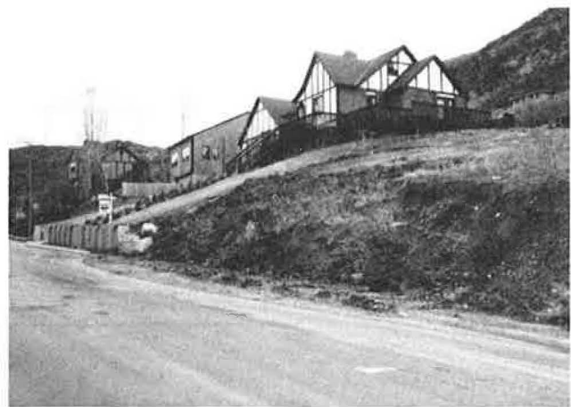
FIGURE 5 View of slide mass with drilled-shaft wall in background.
