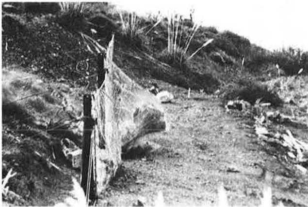
FIGURE 1 Brugg flexible rockfall net in action (rock weighs 3 tons) (Courtesy of John Walkinshaw, FHWA).
