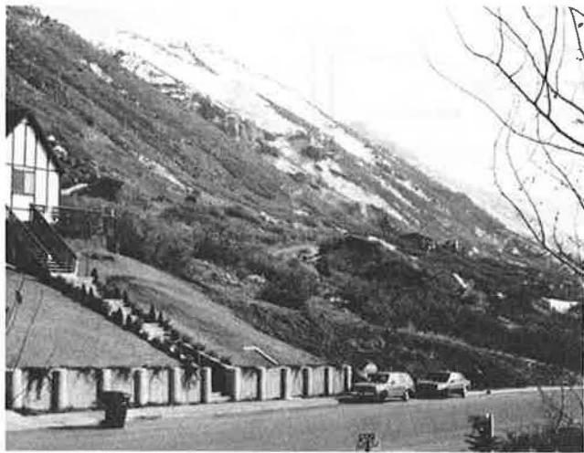
FIGURE 4 View of completed drilled-shaft wall with landslide developing immediately adjacent to it.
