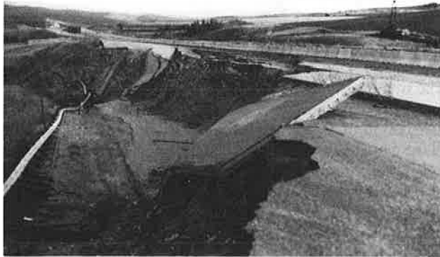
FIGURE 2 View of failed embankment, near Station 297+00, May 1983.
