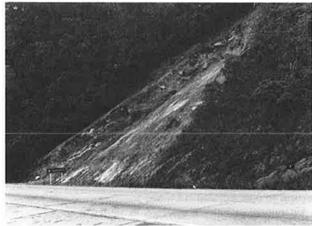
FIGURE 4 Scar of planar slide that partially closed BR 116.
