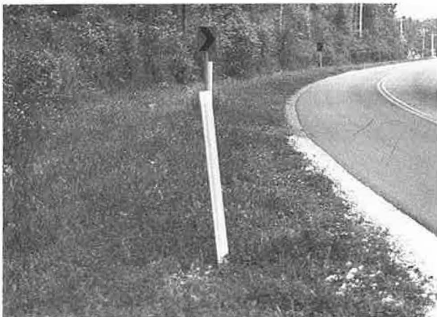
FIGURE 7 Local road containing recycled plastic flexible delineator posts.
