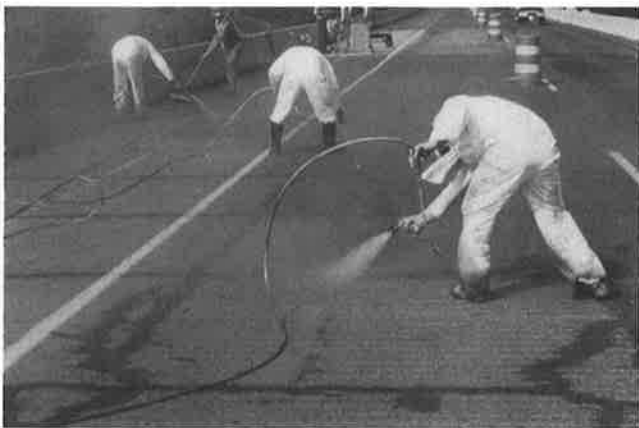
FIGURE 2 Airless spray guns were used to apply HMWM resin to surface of tined bridge deck. Note that work crew is wearing rubber boots and gloves, impermeable coveralls, and canister breathing masks.
