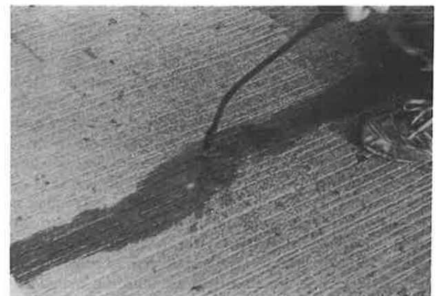
FIGURE 1 HMWM monomer applied to cracks in tined bridge. To maintain good skid number, excess resin in valleys must be broomed over deck surface before it gels.
