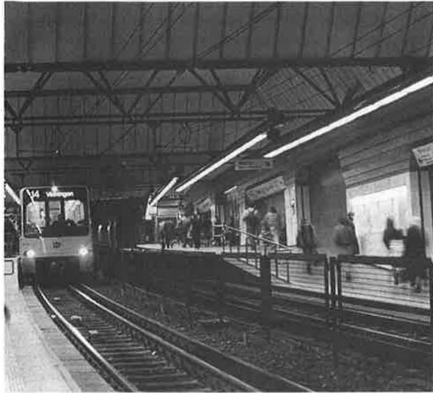
FIGURE 1 LRT underground station.
