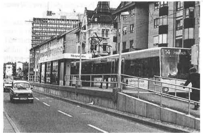
FIGURE 6 High platform at a surface LRT station.
