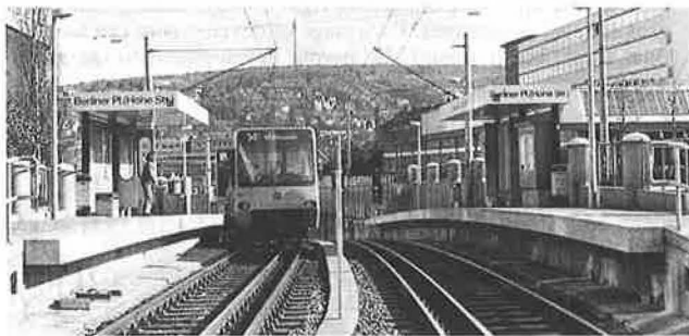
FIGURE 5 Three-rail track for mixed operation.
