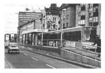
FIGURE 6 High platform at a surface LRT station.
