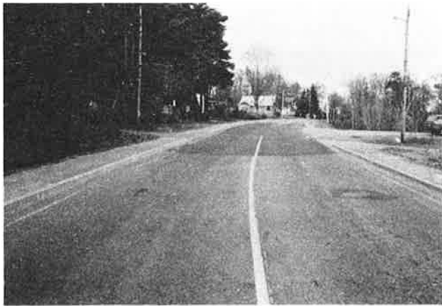
FIGURE 6 Severe differential frost heave of approximately 10-year-old District Road 2 pavement. The extensive padding has been replaced nearly annually to restore surface drainage and ride through the intersection.
