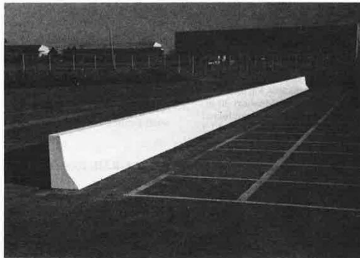
FIGURE 2 Missouri 30-in. New Jersey safety-shape bridge rail.
