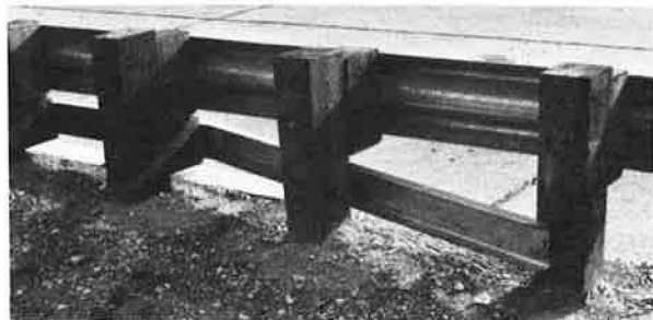
FIGURE 7 Photographs of improved separate end-post transition design test installation.
