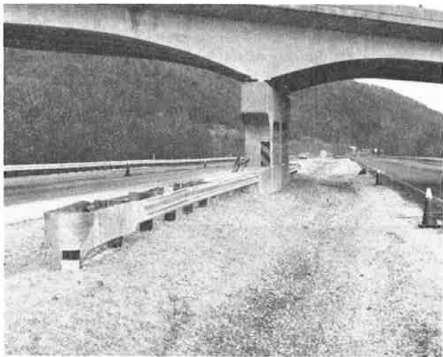
FIGURE 4 CAT installation.
