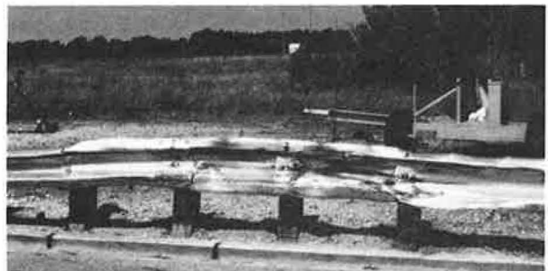
FIGURE 4 Integral end-post transition after Test 3.
