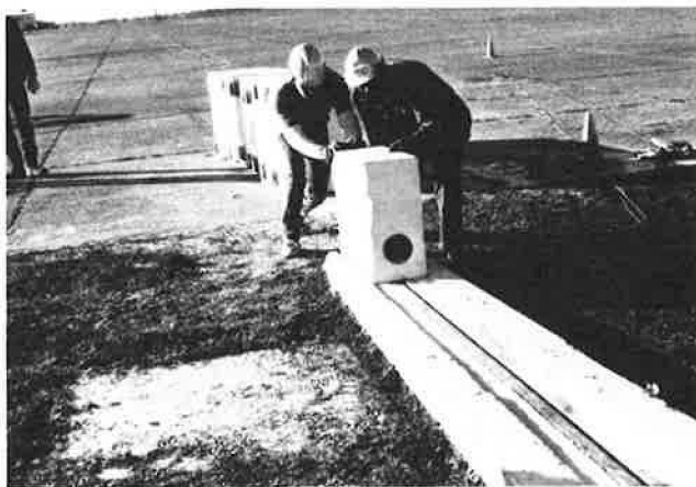
FIGURE 7 Installation of ADIEM terminal modules.
