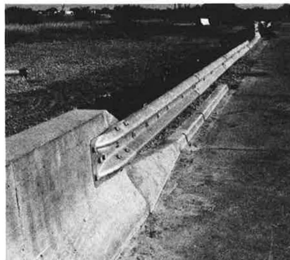
FIGURE 1 Photographs of integral end-post transition design test installation.
