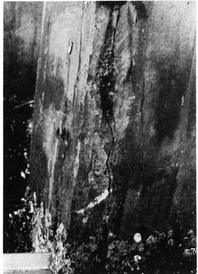
FIGURE 1 Excessive vertical cracking and spalling of concrete in a pile (B. B. McCormick Bridge, Jacksonville).
