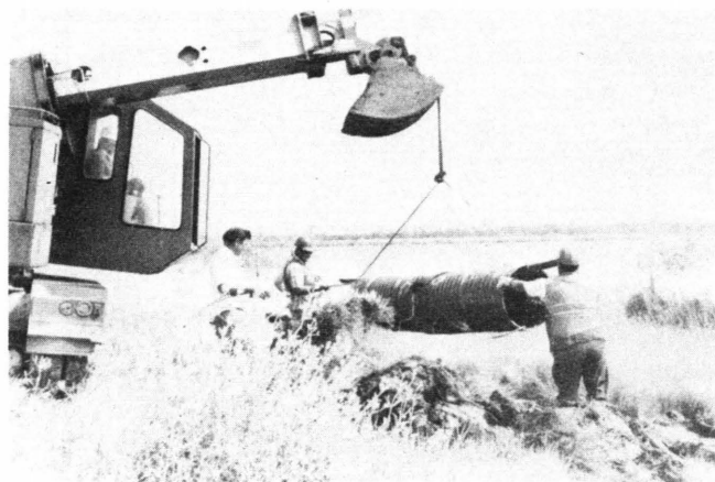
FIGURE 2 One of corrugated steel pipes is lowered into ditch.
