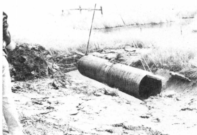
FIGURE 4 Unprotected steel pipe is lowered into ditch.
