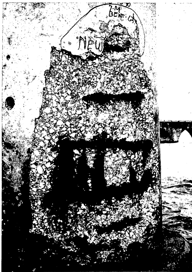
FIGURE 2 Excessive steel corrosion and extensive concrete spalling in a pier (Seven-Mile Bridge, Florida Keys).
