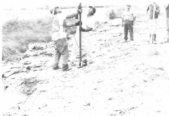
FIGURE 3 External anodes are pushed into ground using Gradall shovel.
