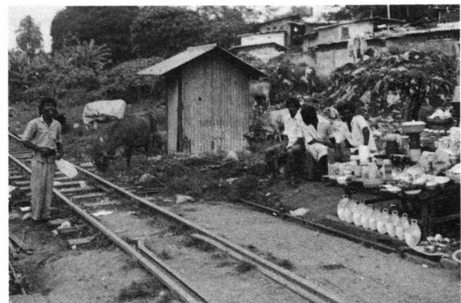
FIGURE 6 Example of encroachment on K.V. rail line right-of-way in Nugegoda.
