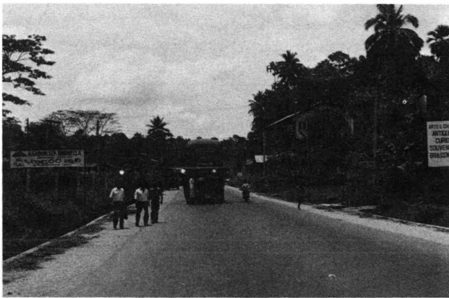
FIGURE 3 Kandy Road; recently reconstructed with adequate lane and shoulder width.
