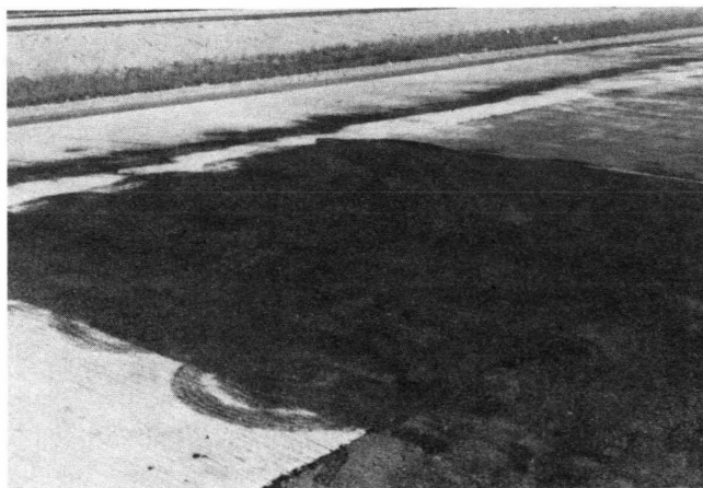
FIGURE 5 Epoxy sealer applied and sanded.
