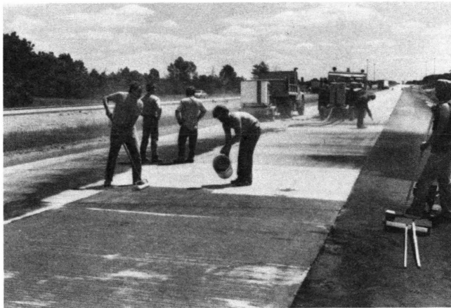
FIGURE 4 Applying sealers, flooding surface, uniformly distributing with roller.
