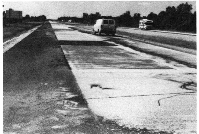
FIGURE 6 Finishing after all sealers applied in traffic lane.
