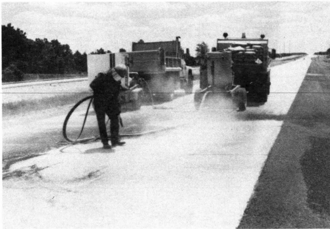
FIGURE 3 Sandblasting operation cleaning the concrete surface, removing the curing compound.
